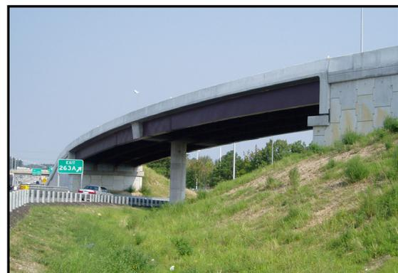
reducing cost and greatly reducing maintenance needs, while also providing graceful sweeping aesthetics. *This is believed to be the first fully-integral curved steel girder bridge in the US.*
