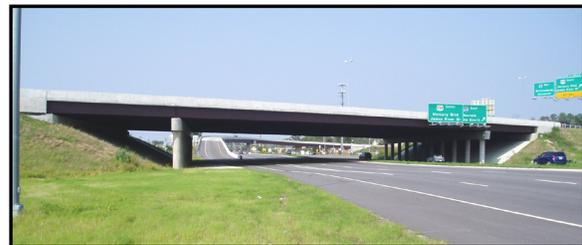
The solution **Alvi Associates** developed is a three-span steel I-girder bridge with a long center span combined with unusually short end spans anchored against uplift by counterweight abutments.
