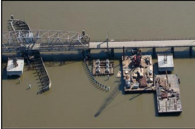
Given that many serious bridge failures have historically been caused by marine vessel collision, the role of **Alvi Associates** was to first perform a comprehensive vessel collision study and then design fender/dolphin systems. The fender system consists of two concrete fenders which guide vessels through the high-level main span, along with providing some collision protection to the bridge. The dolphin system
