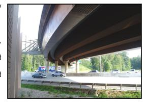
Features include long girder spans, cost-saving high-performance steel, cost-saving radial MSE abutments, and an elegant and unusual capless pier with individual columns supporting each girder.
